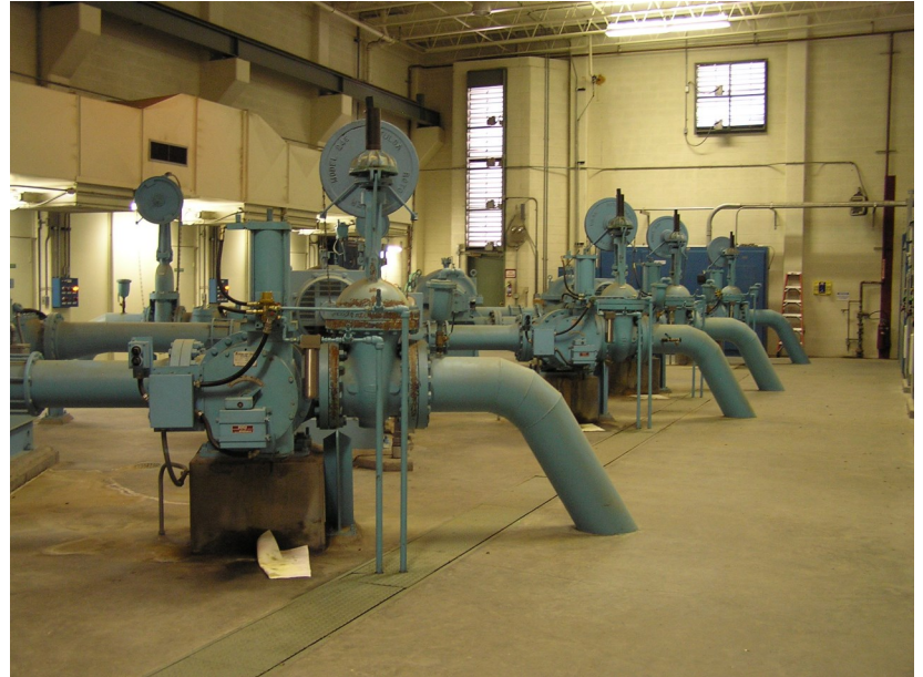
Water pumps for the Fountain Valley Conduit
