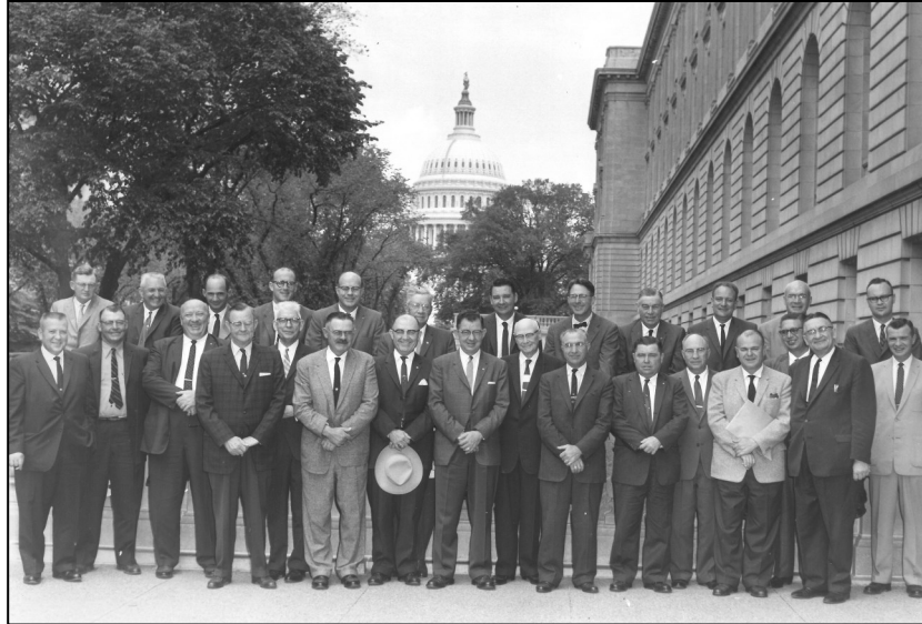
Arkansas Valley community leaders traveled to Washington, D.C., to promote the Fryingspan-Arkansas Project.
