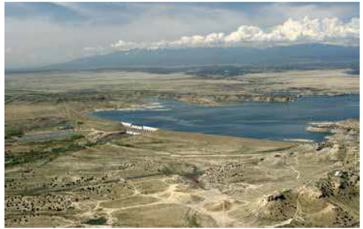
Pueblo Dam and Reservoir, which were constructed for the Fry-Ark Project.
