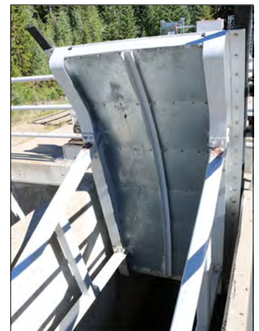
Cunningham Diversion gate.
