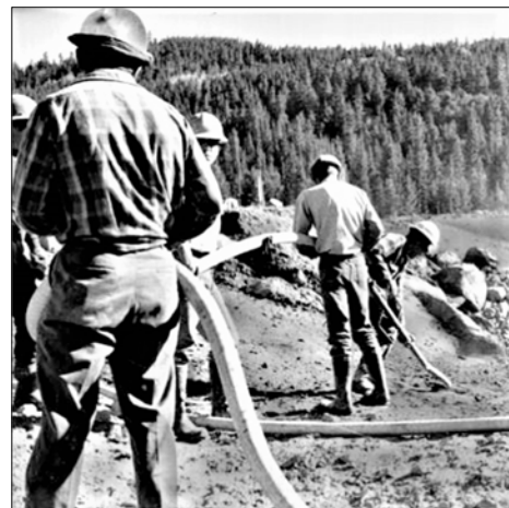
Construction of Sugar Loaf Dam at Turquoise Reservoir. (Reclamation Photo)
