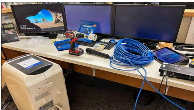
Audio-visual upgrade in progress in the Board Room.
