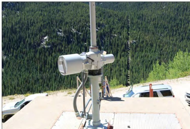
Gate actuators, such as this one at the Granite Syphon, were installed in the past few years. The remote operation reduces the time needed for Reclamation workers to travel to a site and manually open and close the gates. (SECWCD photos)
