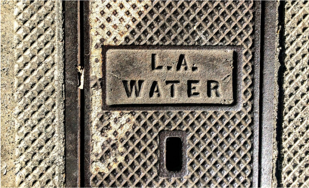
A water meter cover in Los Angeles, California. Photo © J. Carl Ganter/Circle of Blue
