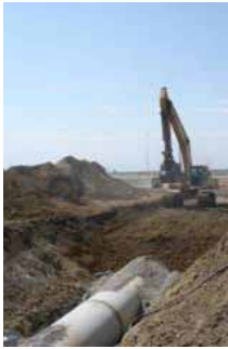
Reclamation sample picture of Conduit construction.
