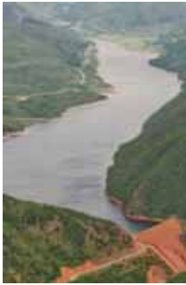
Ruedi Dam and reservoir was completed in 1968.
