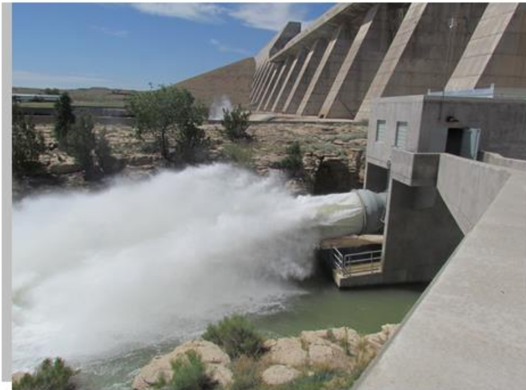
Pueblo Reservoir North Outlet
