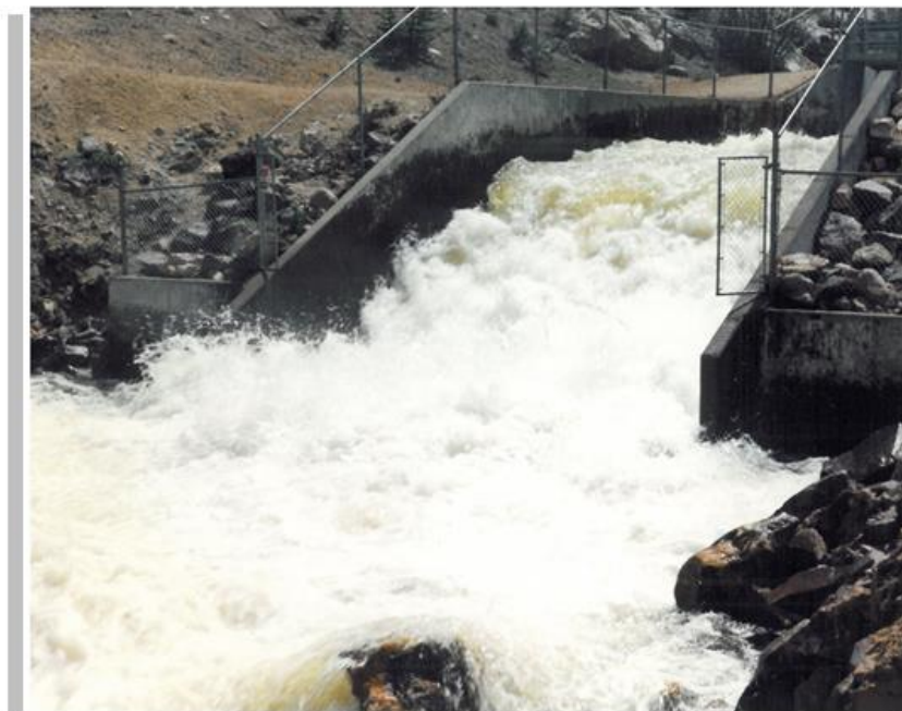
Outlet of Boustead Tunnel
