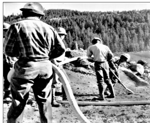
Sugarloaf Dam construction in the 1970s.
