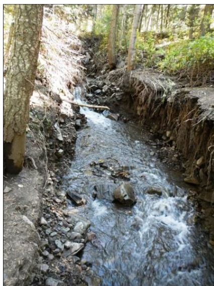
Erosion at the burn scar from the 2016 Hayden Creek fire in Fremont County.
