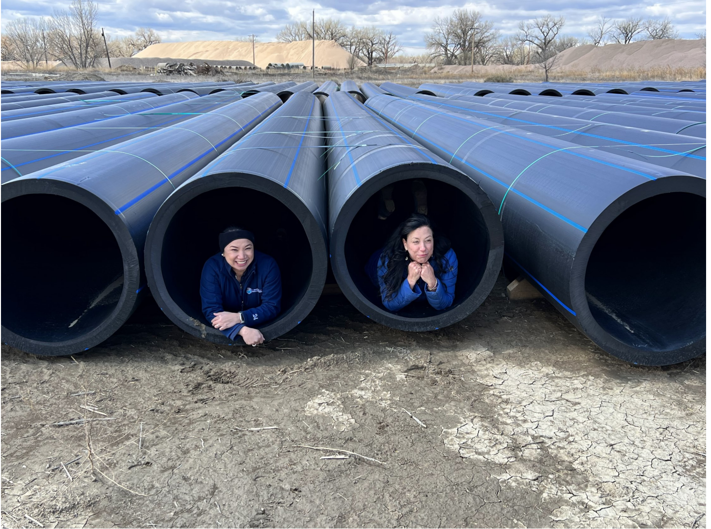
Bureau of Reclamation Commissioner Camille Calimlim Touton and Colorado Water Conservation Board Executive Director Becky Mitchell celebrate the beginning of construction on the Arkansas Valley Conduit on Friday, April 28, 2023. Photo by SECWCD
