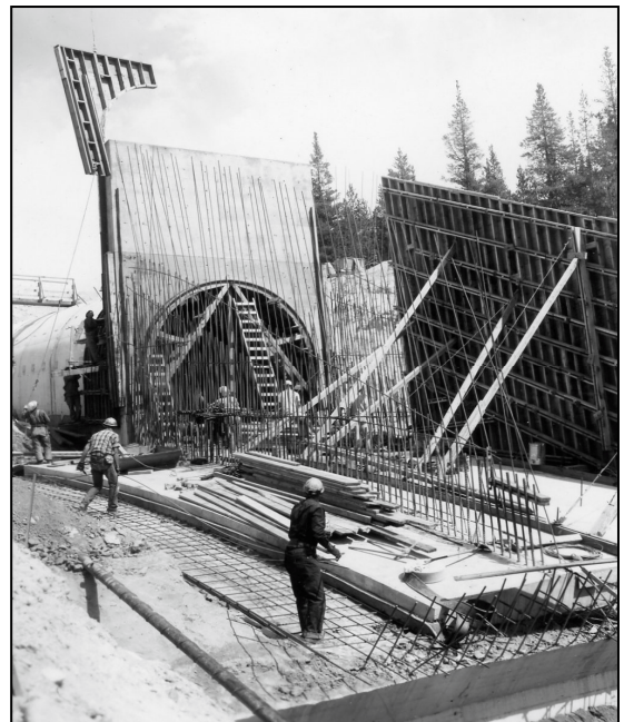
Ruedi Dam Construction during the 1960s
