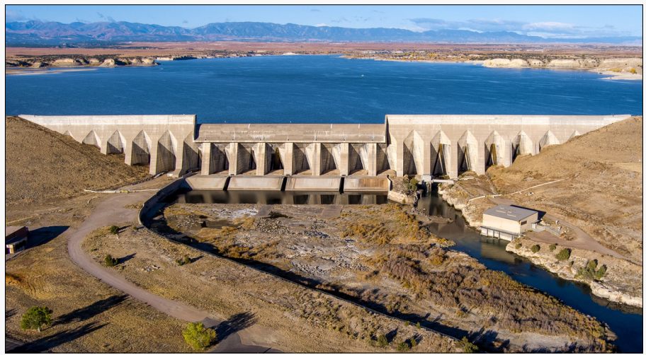
Pueblo Reservoir provides terminal storage for the Fry-Ark Project. The James W. Broderick Hydropower Plant is on the right. (Mike Sweeney photo)
