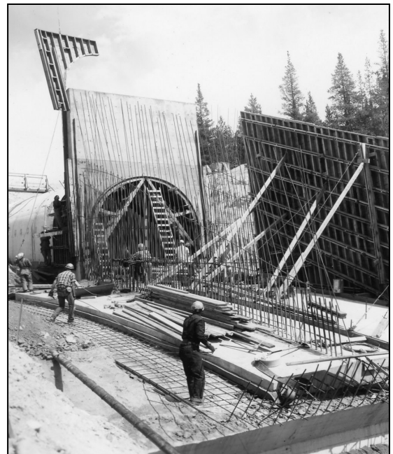
Ruedi Dam Construction during the 1960s
