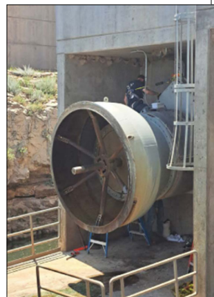
Stripped thrust nuts on the Pueblo Dam cone valve were repaired in August by Reclamation. (Reclamation photos)
