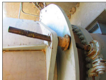
Stripped thrust nuts on the Pueblo Dam cone valve were repaired in August by Reclamation. (Reclamation photos)
