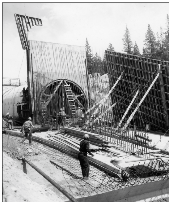
Ruedi Dam Construction during the 1960s
