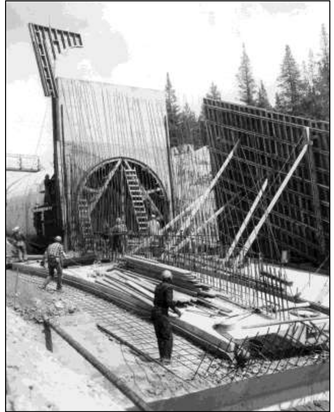
Construction at Ruedi Dam during the 1960s
