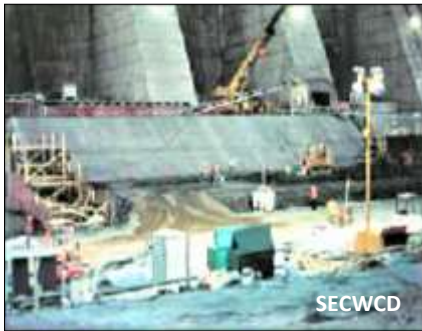
Work on Pueblo Dam in 1998
