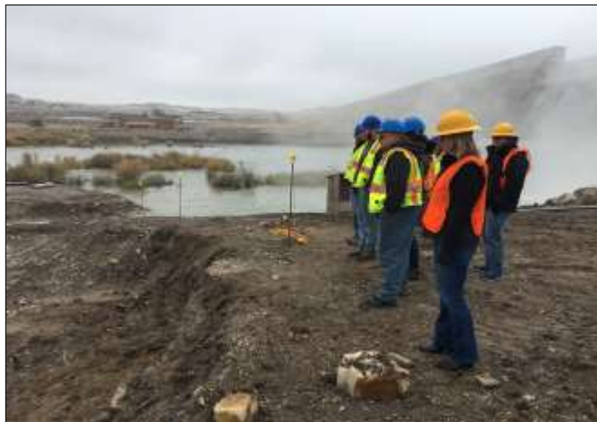
District staff arranged a tour of the Pueblo Dam hydro site for Colorado Water Conservation Board staffers in November. CWCB is funding the construction loan.
