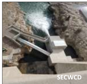
North Outlet Works
