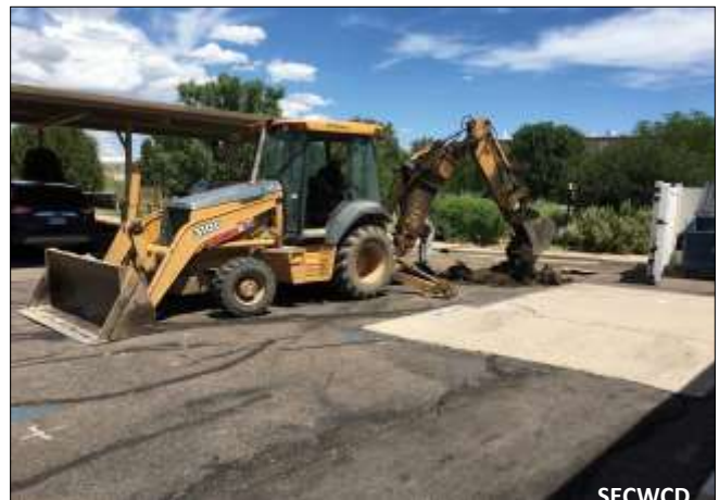
Minor repairs occurred in the District parking lot in July.
