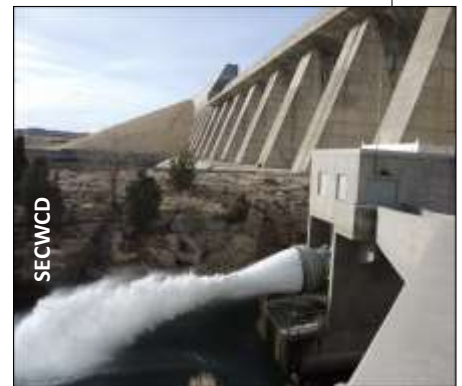
North Outlet Works at Pueblo Dam.
