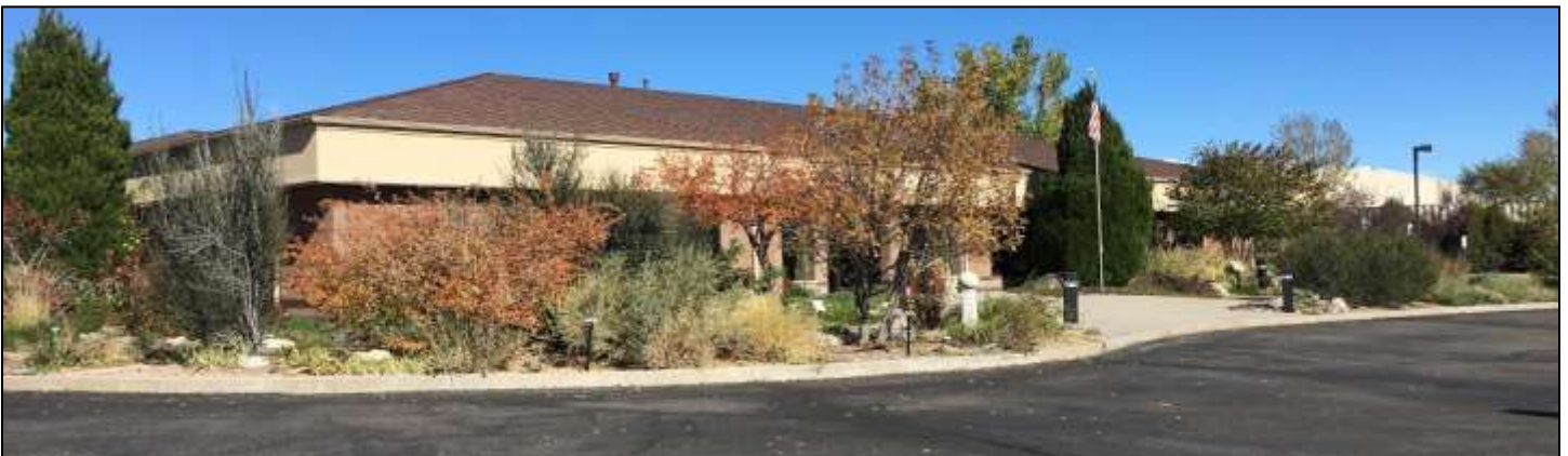
Southeastern Colorado Water Conservancy District offices at the Pueblo Memorial Airport Industrial Park
