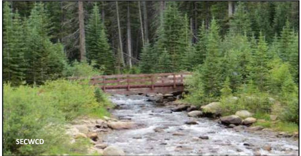
Water flows in Hunter Creek, part of the West Slope collection system of the Project.
