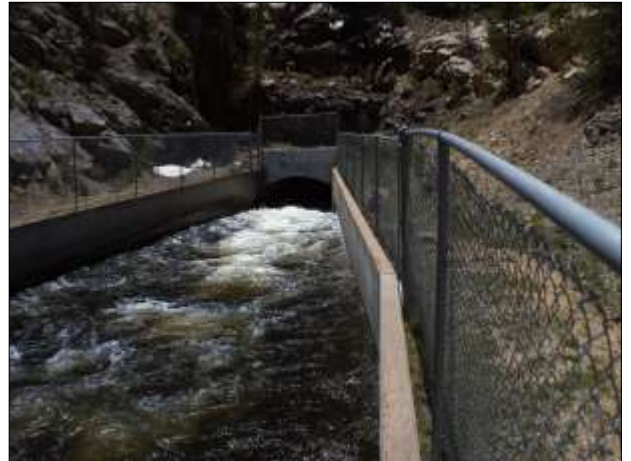
Water flows through the Boustead Tunnel
